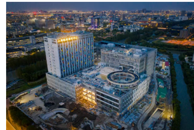
The research hospital under construction.
